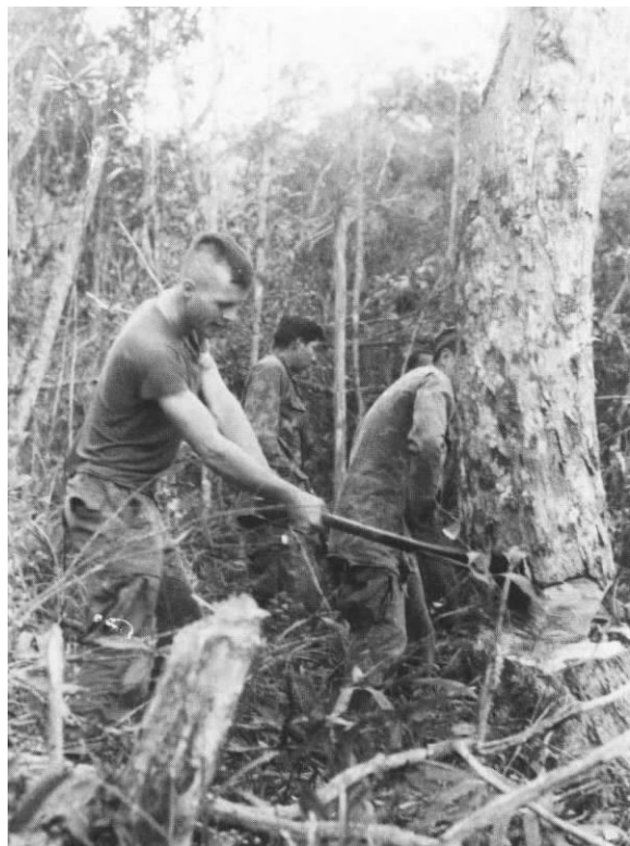
Abel Papers, Marine Corps Historical Center Engineers accompanying the 9th Marines clear a landing zone for resupply and medical evacuation helicopters in heavily wooded terrain south of Vandegrift.
